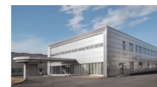
Fukaya Center, R&D Division
