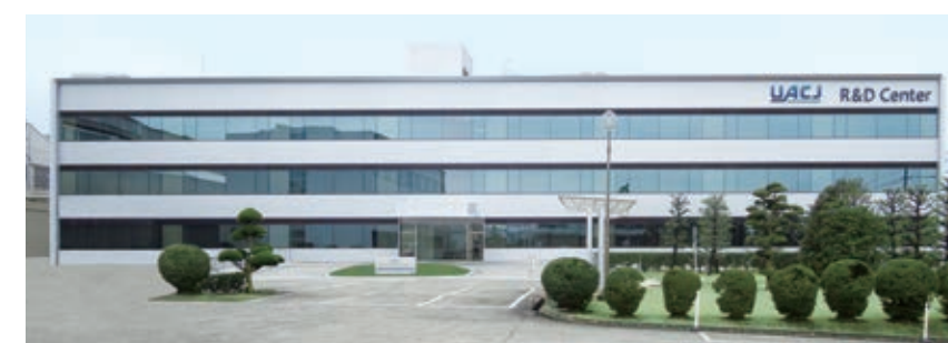
The R&D Center after renewal. Aluminum honeycomb panels are used for the exterior.
