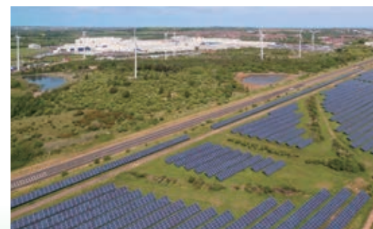
Solar panels at Nissan's Sunderland plant (UK)
